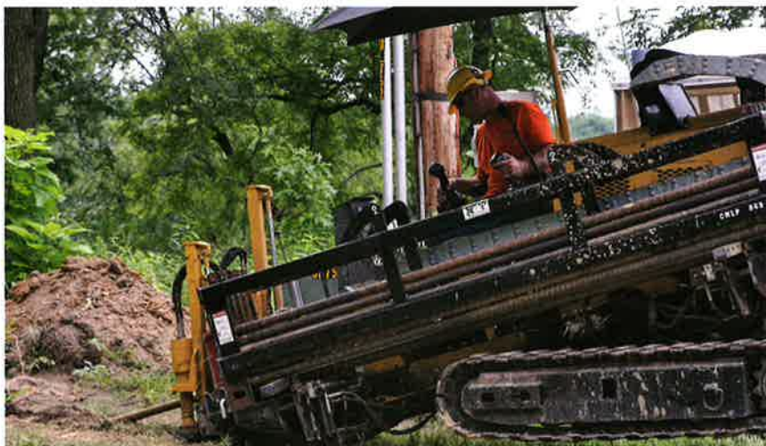
Installation of a closed-loop geothermal system.
